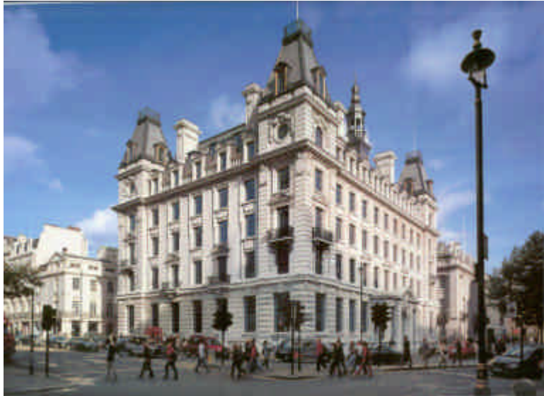
London - Office Fit Out
