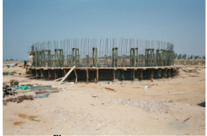
CASS™ SBR Basin under construction
